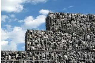
Fig. 1: Typical Gabion Wall Structure.
